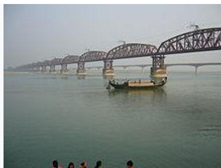
Hardinge Bridge , Bangladesh, crosses the Ganges-Padma River. It is one of the key sites for measuring streamflow and discharge on the lower Ganges.
