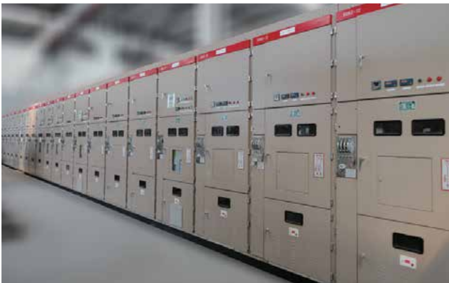
• High Voltage Distribution Cabinet
