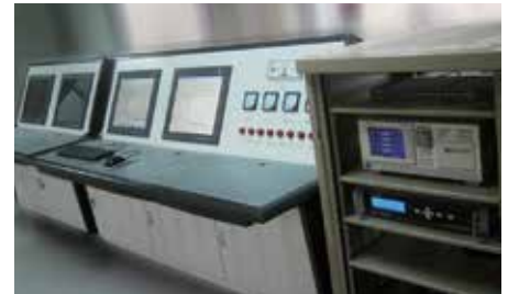
• Central control room
