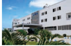
Rudrapur Plant (Green Building)
