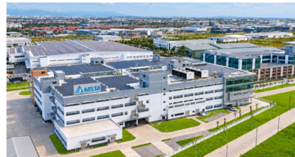
Delta Thailand BP5 Plant
