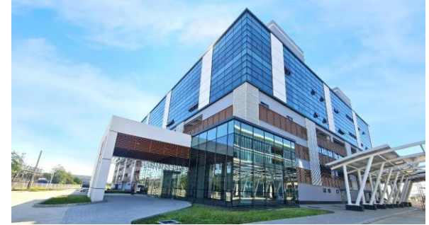
Delta Thailand BP5 Plant
