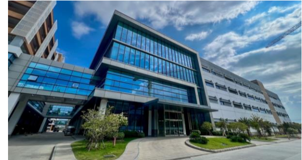
Delta Thailand BP8 Plant
