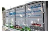
2MW/1MWh Energy Storage System for Xia Xing Power Station on Kinmen Island
