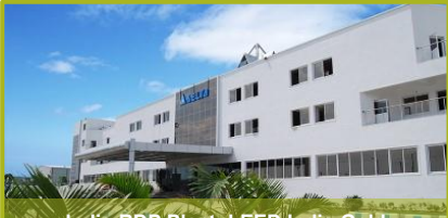
India RDP Plant, LEED India Gold
