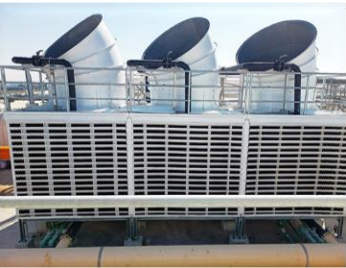
Cooling Tower in HVAC System
