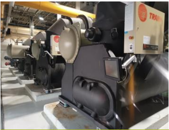
High Eff-Chiller for HVAC System
