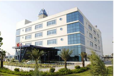
India Gurgaon Plant
